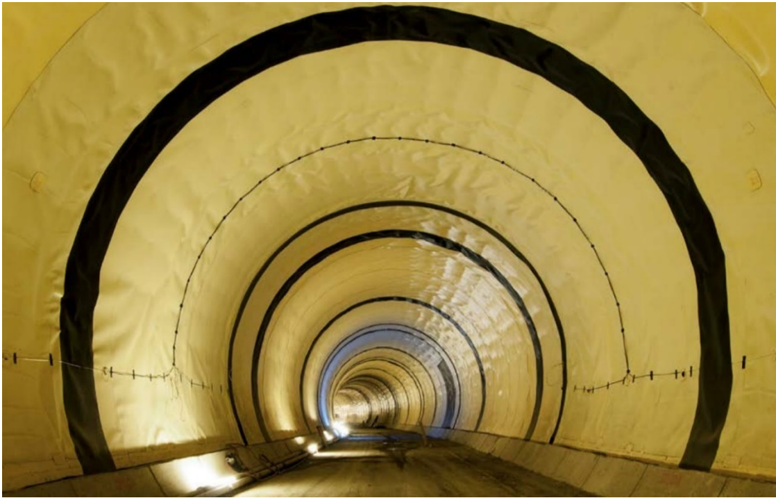
Figure 11-2 Installed water proofing membrane
